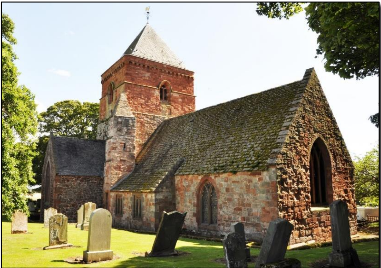
A view from the northwest.
