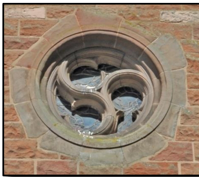
I have not found many mouchette windows in English Saint Botolph churches, and I was particularly pleased to spot this triple mouchette on the south face of the south transept.
