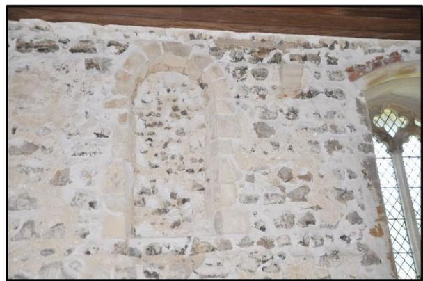
and the other from the outside of the north wall. Both window slits are actually the same size although due to the splaying within the fabric of the wall, the most westerly (viewed from the interior) looks much larger.
