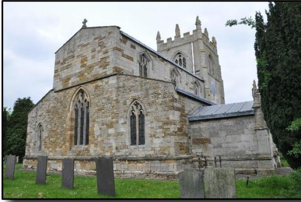
With the exception of the chancel (which is ironstone) the church fabric is of limestone. This suggests that the chancel might have been added during the restorations of C19 but at present I can find no record of this. The fine but massive C13 arches which support the central tower are the oldest part of the church.
